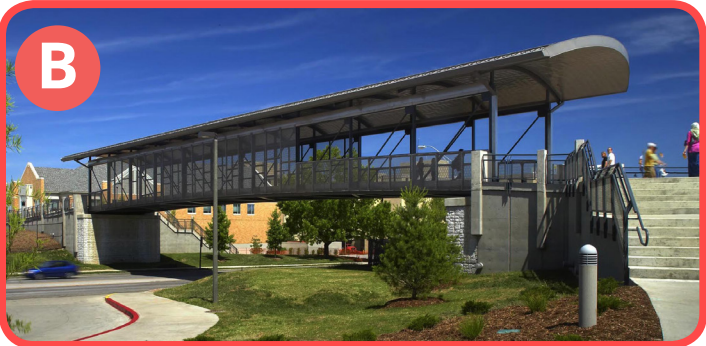
University of Missouri Pedestrian Bridge
