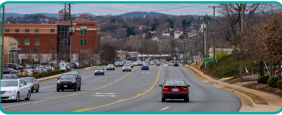
Route 250 facing west.
